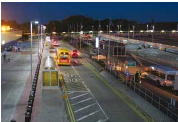
The Aberdeen airport forecourt at full illumination
